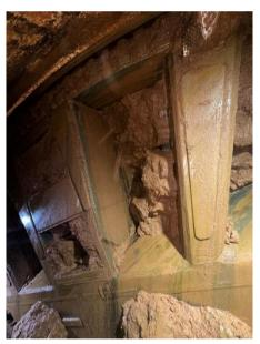
The photograph shows Sidmouth Formation Weathering Grade I/II of Mercia Mudstone Group, as exposed through the Tunnelling Boring Machine (TBM) cutterhead, during a maintenance intervention of the Bromford Tunnel Project.
